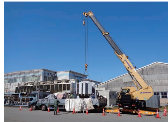
PCB waste removal operations
