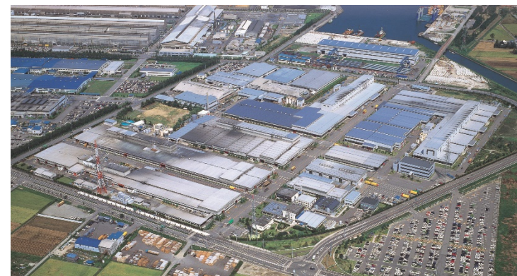
*1 Overview of the Imizu Plant
