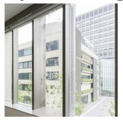
Natural ventilation windows for commercial buildings and apartments. "Swindow" automatically opens and closes with the wind (left).
