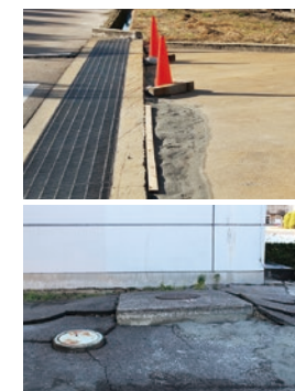
Nago Plant (Ground protrusion and liquefaction)
