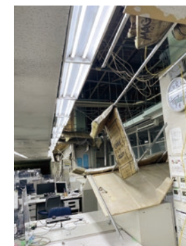
Takaoka Plant (Fallen ceiling material)
