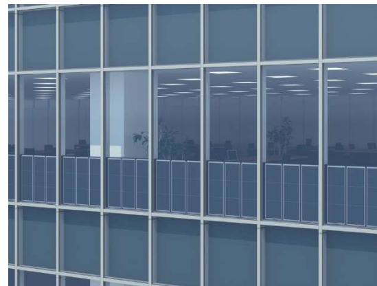
Units installed in a high-rise building (for illustration purposes only)
